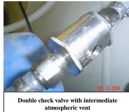
Double check valve with intermediate atmospheric vent
